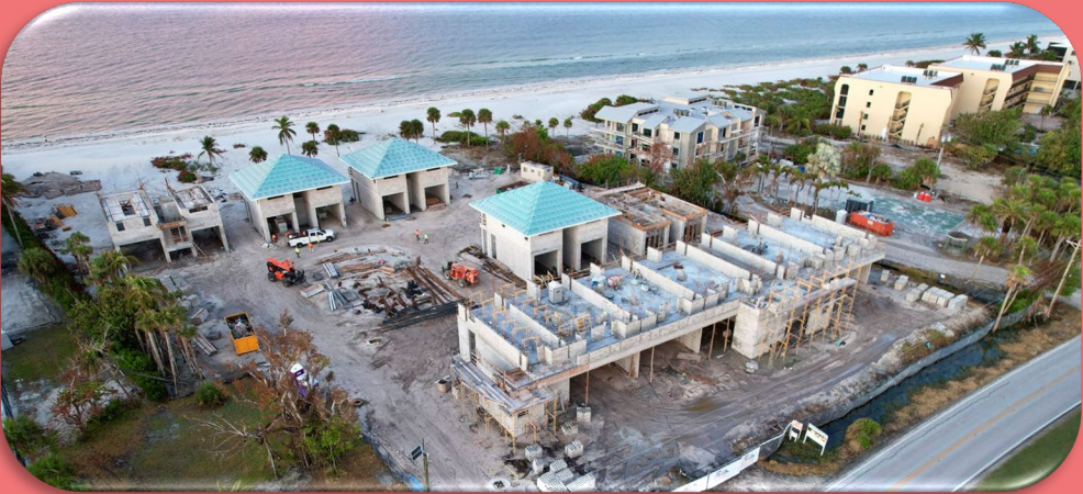
Construction as of 10-31-2024
